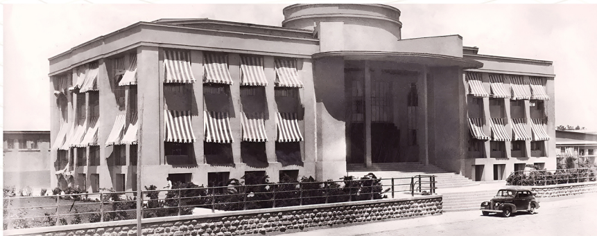
Iran Tobacco Company Building Tehran _ Qazvin Street _ 20 October 1937 (Opening Day)
